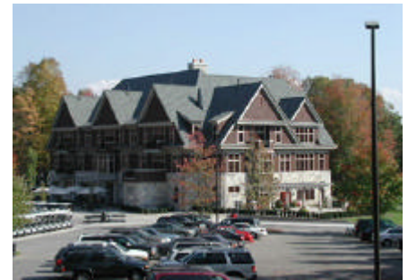
The New Kinlochen Lodge & Pro Shop
